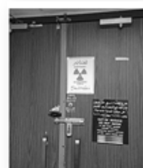
Figure 18. Access door Locking system.
